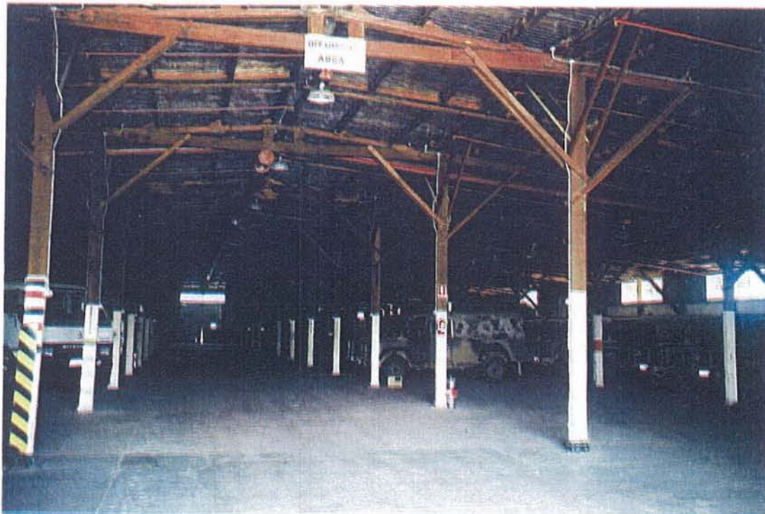
Fig. 3.8 INTERIOR OF A TYPICAL TIMBER POSTS AND BEAM STOREHOUSE AT NORTH BANDIANA, SHOWING SIMILAR TIMBER CONSTRUCTION TO THAT FOUND AT DN3DC
