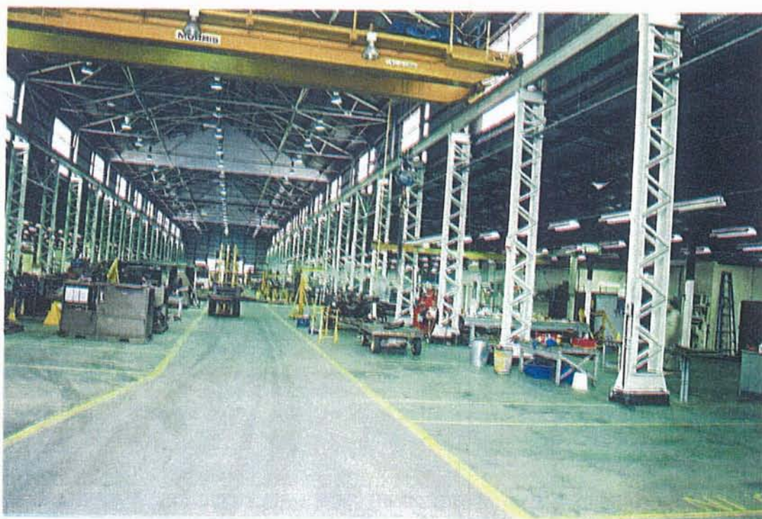
Fig. 3.2 INTERIOR OF BUILDING 9, A WORLD WAR II COMPOSITE TIMBER AND STEEL FRAMED STORE BUILDING
