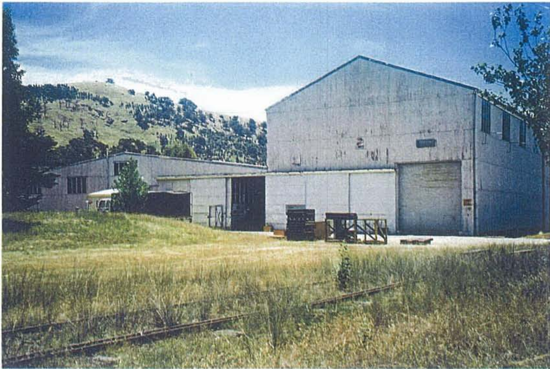
Fig. 3.9 TYPICAL EXAMPLE OF THE FOUR STOREHOUSES AT NORTH BANDIANA, WHICH COMPRISE OF A LOWER TIMBER WING, AND A RAISED STEEL FRAMED WING WHICH STRADDLES THE RAILWAY LINE
